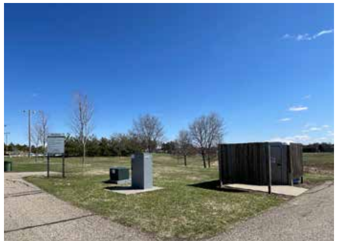
Restroom Enclosure & Electrical Cabinets
