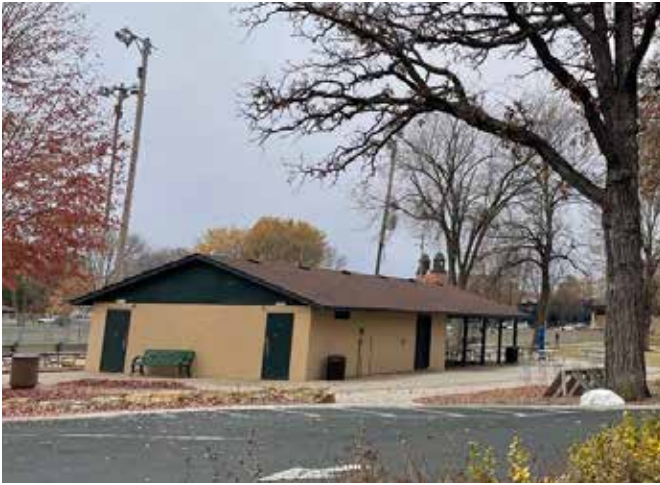
Restrooms & Picnic Shelter
